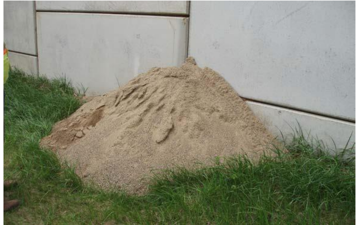
Backfill Leakage
